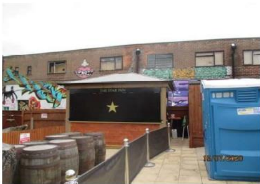
External bar with warehouse to Moore Gate in the background
